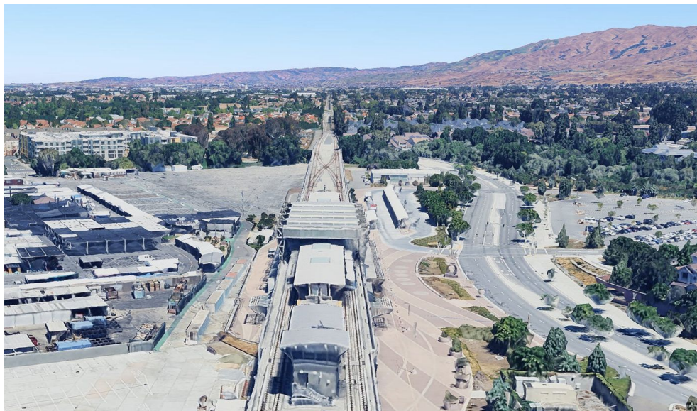
Berryessa Station in San Jose.
